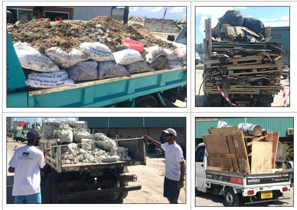
Figure 38: (a) Soil and rock in polypropylene sacks (b) truck overflowing with wooden pellets and other mixed waste (c) Large pieces of demolished concrete (d) Truck overflowing with mostly wooden pellets with some metal containers on top.
